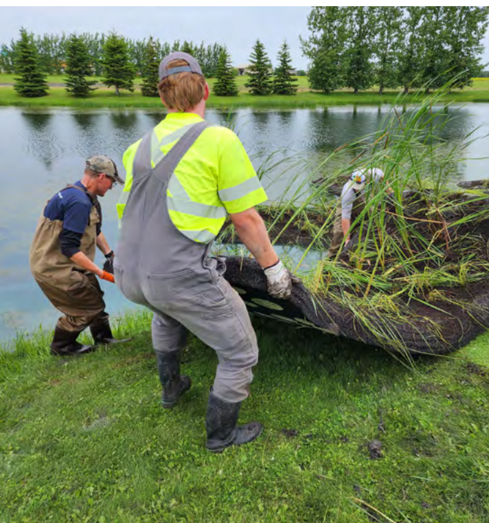
In Springfield, Manitoba, IISD and local municipality staff install floating wetlands on a retention pond to improve water quality and remove contaminants. (Joey Simoes/IISD)
